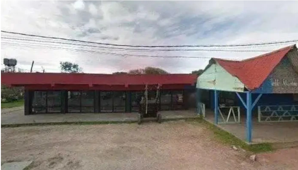
Karamba chiveteria street view y 360
