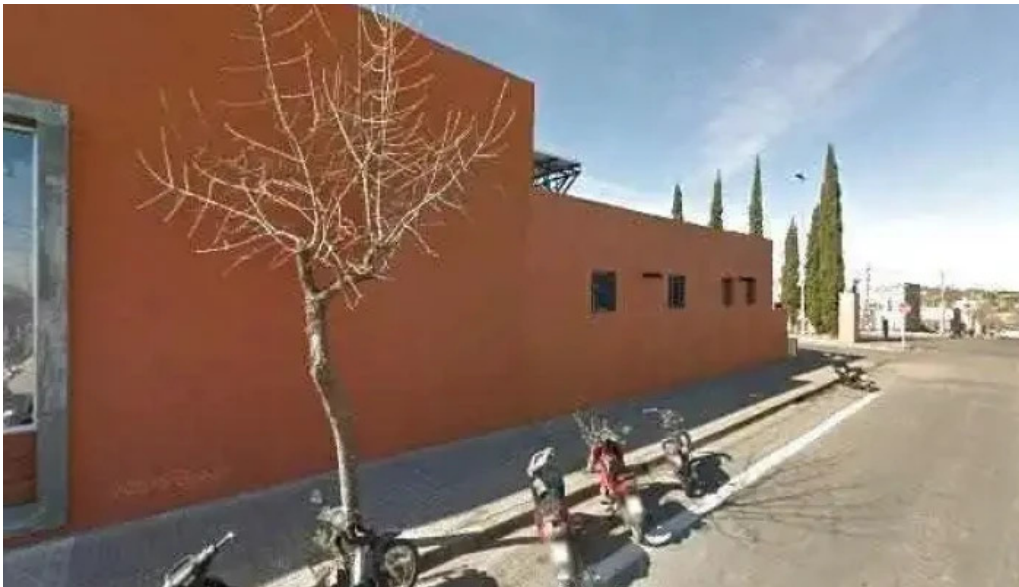
Subway street view y 360
