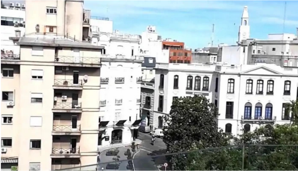
Alma historica boutique hotel exterior
