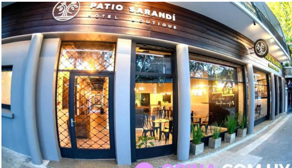
Patio sarandi exterior
